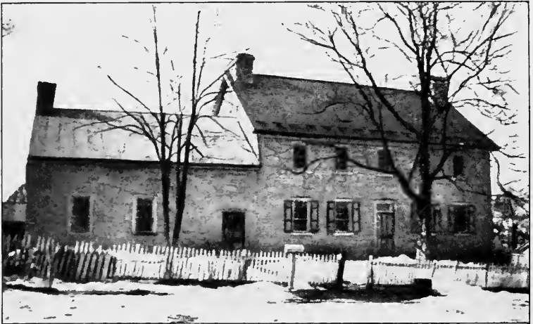
Old Poe Farmhouse—East View
